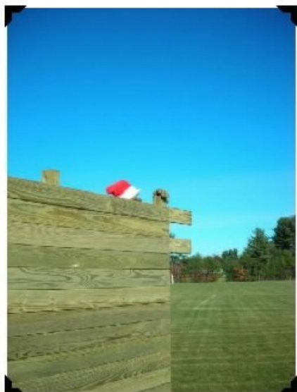
Figure 38 - Decking Construction - November 24, 2007
