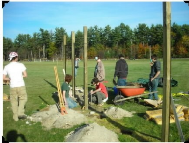
Figure 33 - Post Erection November 3 & 4, 2007
