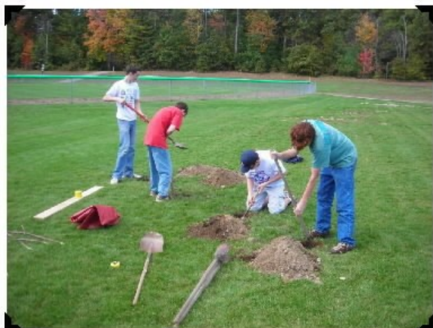
Alec, Matt, Max and Nick making progress on the post holes
