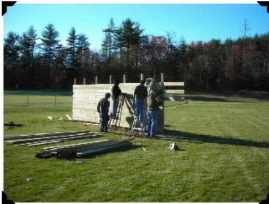
Figure 36 - Decking Construction - November 23, 2007
