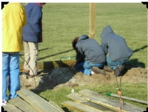
Figure 35 - Decking Construction - November 23, 2007
