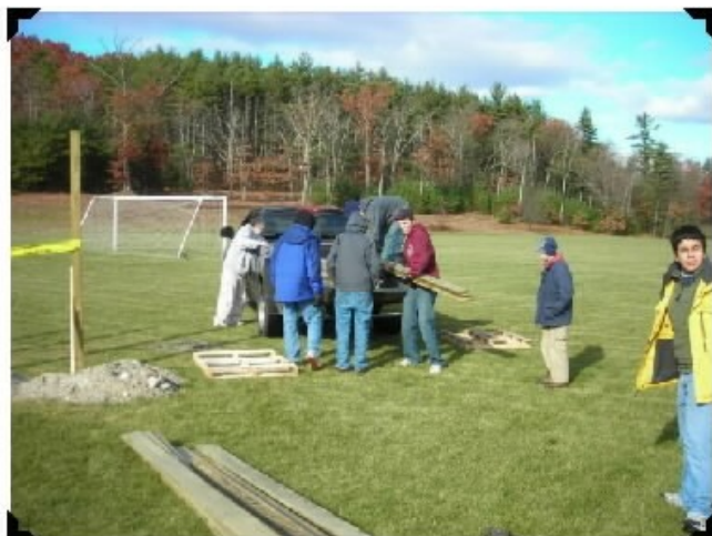
The crew unload the decking from Mr. Pinque truck.
