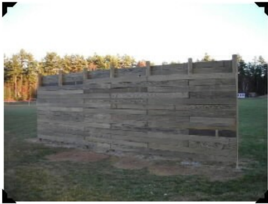
Figure 37 - Decking Construction - November 23 & 24th, 2007
