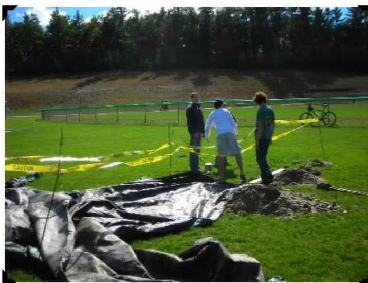
Post Hole Digging Completed!
